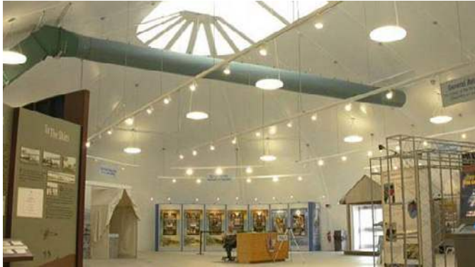
Interior of tension membrane structure
